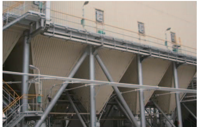
Electrostatic Precipitators (EP)
