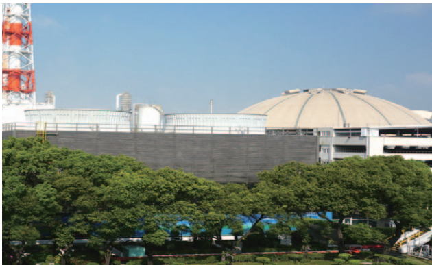
Linyuan Public Utilities Plant
