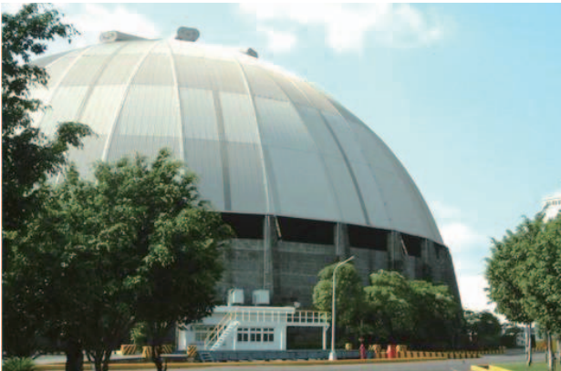
Indoor Coal Yard with Closed Delivery System
