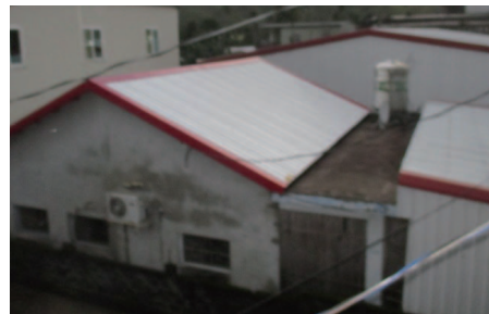
After Renovation - New Roof
