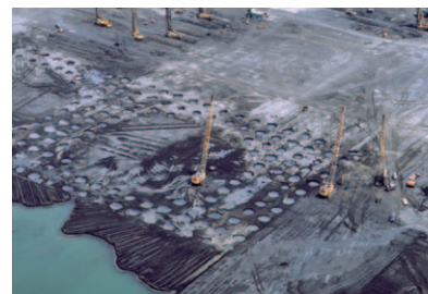
Land Reclamation of No.6 Naphtha Cracking Project
