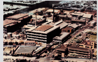
Aerial Photograph of Kaohsiung Plant
