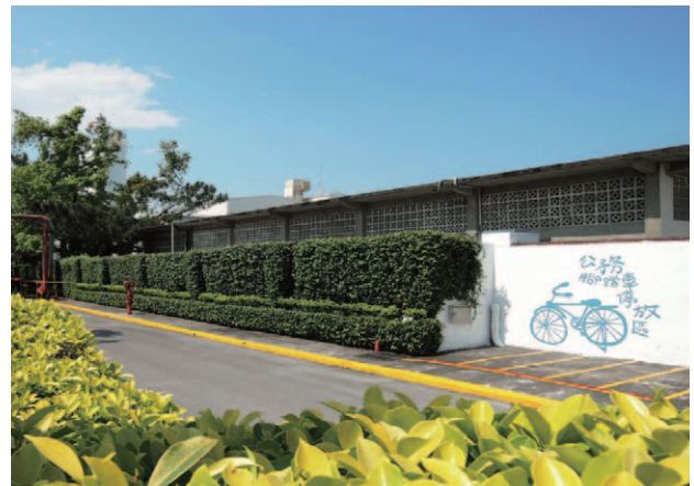
Tungshan Carbide Plant
