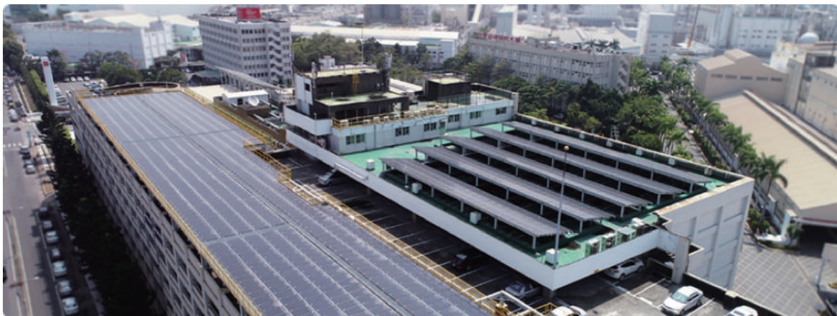
Solar Power Generation System at the Renwu Complex
